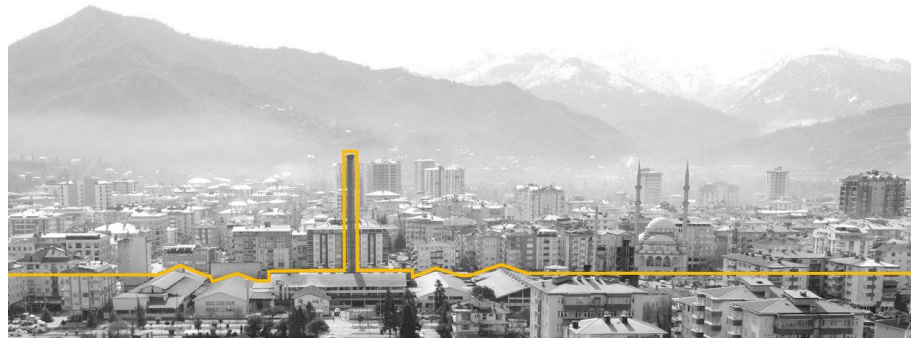
Figure 5. Arhavi Tea Factory chimney (authors' archive)
