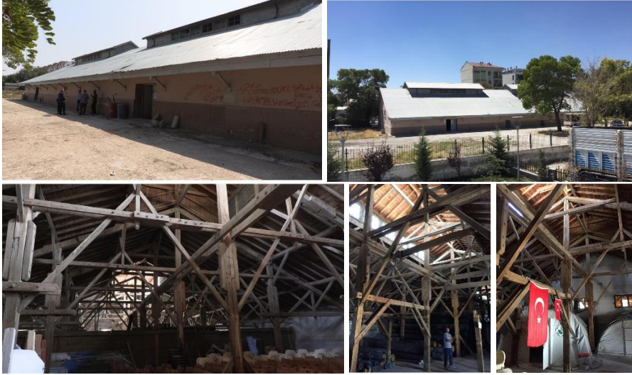
Figure 2. The Karapınar Grain Warehouse before restoration (Konya Metropolitan Municipality archive).
