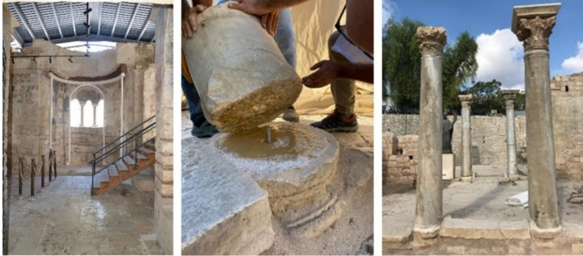
Figure 30. Reinforcement of SEC I dome drum and completion of columns (AMoCT-PR-4)
