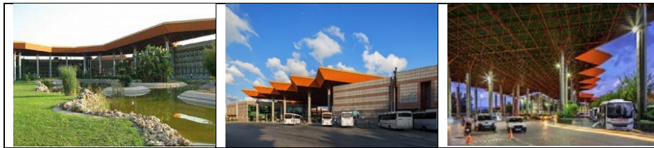
Figure 2. Antalya bus station eaves and broken plaque design (URL 1)
