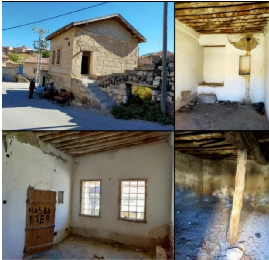
Figure 19. The old house investigated in Emmiler.
