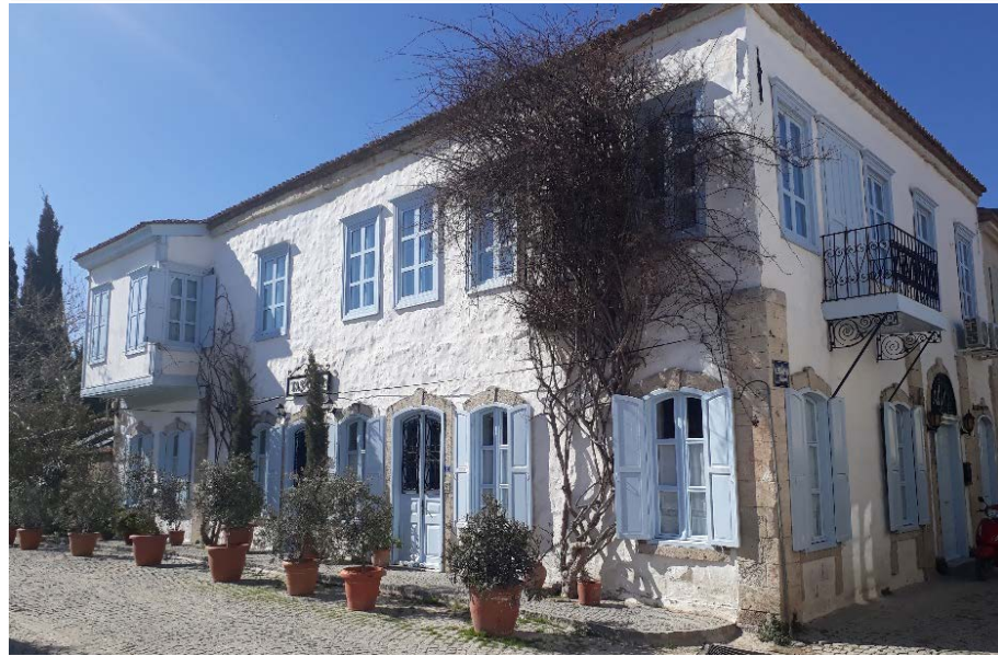
Figure 5. Bay window of Building 2
