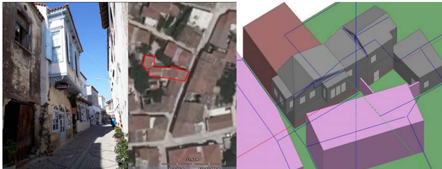
Figure 1. Photo, satellite view and energy model of the Building 1 (Google Earth, 2017)
