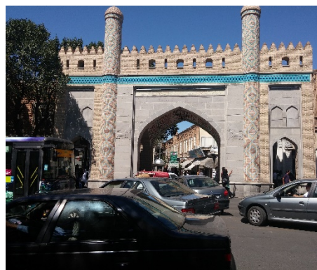
Figures 6. Old-style facades and the special architectural pattern (left)
