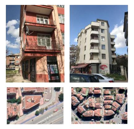
**Figure 13.** Building layouts with nonparallel axes
