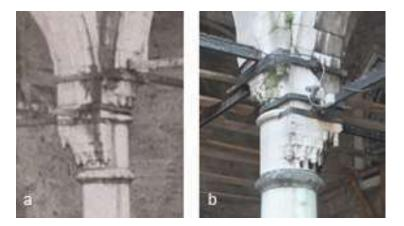
There are two iron bracelets on the upper capital. Figure 16 shows that these bracelets in the CL1 existed in the late 19th century - early 20th century. They have been added in a repair before this date. The last repair of the mosque was made between 2013 and 2015. During this restoration, the surface was cleaned, iron tie rods were cleaned and painted, and cracks were repaired by injection (Figure 15).
