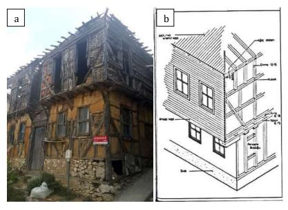
**Figure 27.** a) The building located at Hamamdere Street no: 44 (*Photo; Aydın, 2017*). b) Construction techniques and materials in wooden structures (*Teker, 1992, p. 45; Table 9*).
