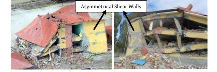
The location of shear walls should be chosen carefully, keeping in mind that the centers of gravity and rigidity are supposed to be as close together as possible. If the shear walls are concentrated on one side of the building, there will be excessive torsional eccentricity and uneven displacements in the structure (Ozmen & Unay, 2007), and shear walls can be responsible for excessive damage during the earthquakes, as observed in the school building.
