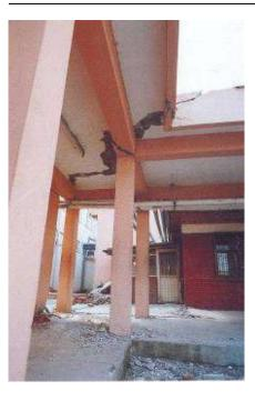
**Figure 3.** Damage in the re-entrant corner of an L-shaped building (source: Anonymous, 2000, Arslan and Korkmaz 2007)
