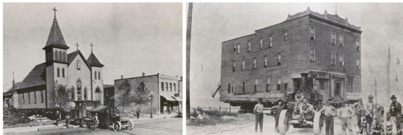
Figure 46., 47. Moving the buildings made of different materials and used with different functions in the city of Hibbing (Fisher, 1971; Curtis, 1979)
