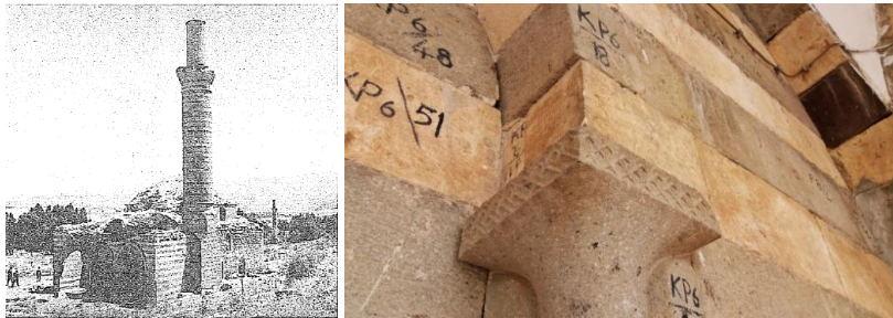
Figure 14., 15. The state of the Baysungur Mosque before the moving (Danık, 2004) and the numbering of its stones during the transportation process (Parlak, 2004).
