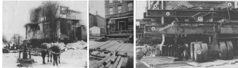
Figure 19., 20., 21. Examples of equipment used in traditional and modern methods of moving historical buildings (Goblet, 2006)
