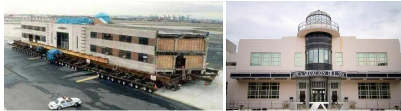
Figure 50., 51. Transporting process of the terminal building (URL 10)
