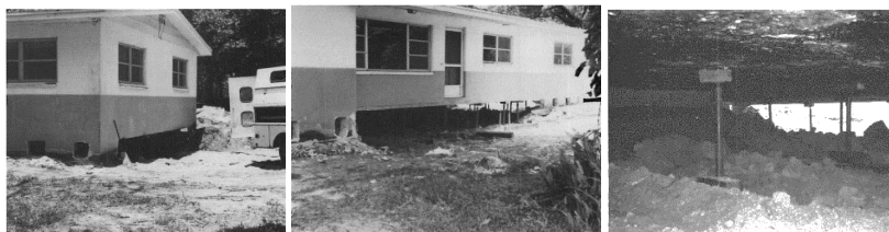
Figure 16., 17., 18. The process of separation from the foundations of the structure (N.F.P.C., 1990)
