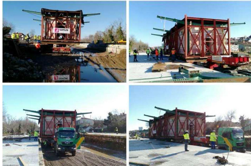
Figure 57., 58., 59., 60. Transporting process of Yeşilköy Train Station Building (URL 9, URL 10)
