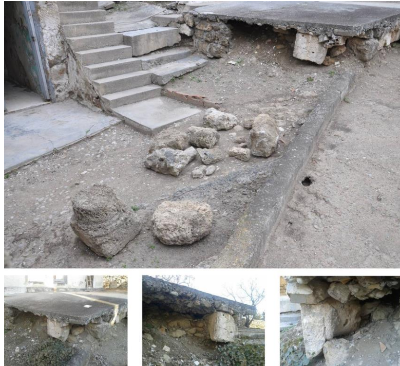
Figure 24. Image of the antique column base under the concrete platform
