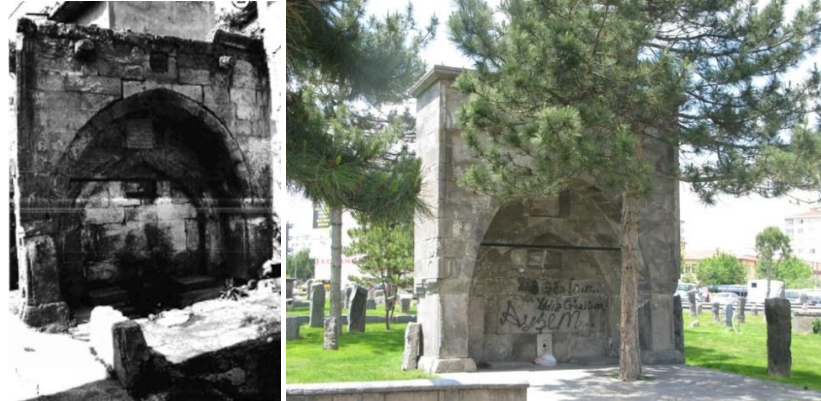
Figure 10., 11. View of Hacı Mehmet (Kaptan Pasha) Fountain before moving (Archive from K.K.V.K.B.K.) and its location in Seyyid Burhaneddin Cemetery (Batukan, 2017)
