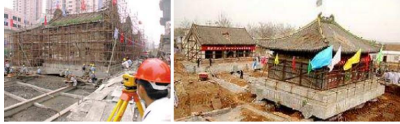
Figure 40., 41. Transporting process of Jinlun City Hall and Quyuan Temple (Lu ve diğ., 2010)
