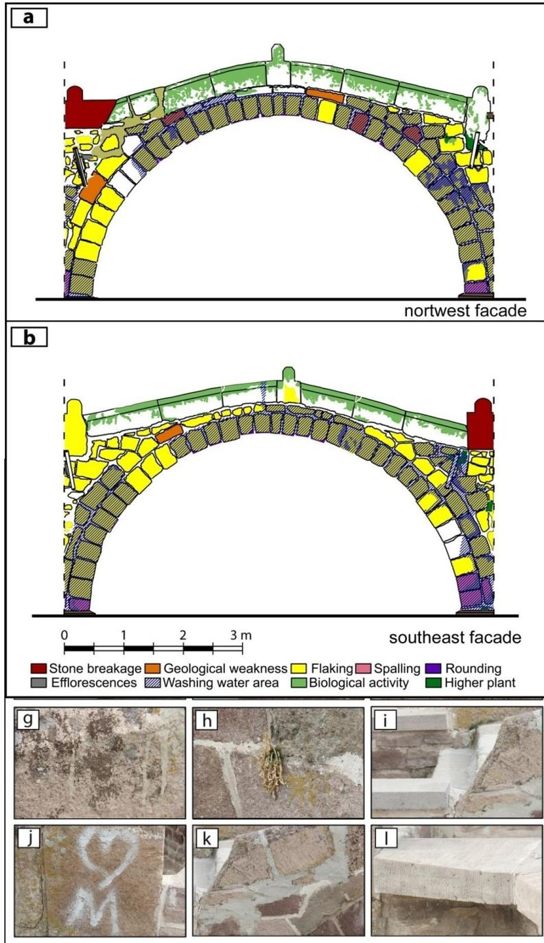
**Figure 8.** Deterioration views in the Mısırlıoğlu Bridge; a) spalling, b) rounding, c) flaking, d) geological weakness and rounding, e) efflorescence, f) fissure, g) biological activity, h) higher plant, i) stone breakage, j) graffiti, k) cement based mortar, l) unoriginal stone.
