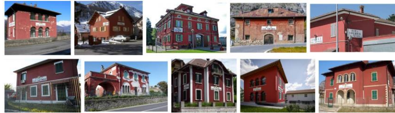
Figure 4. Architectural features of ANAS houses.
