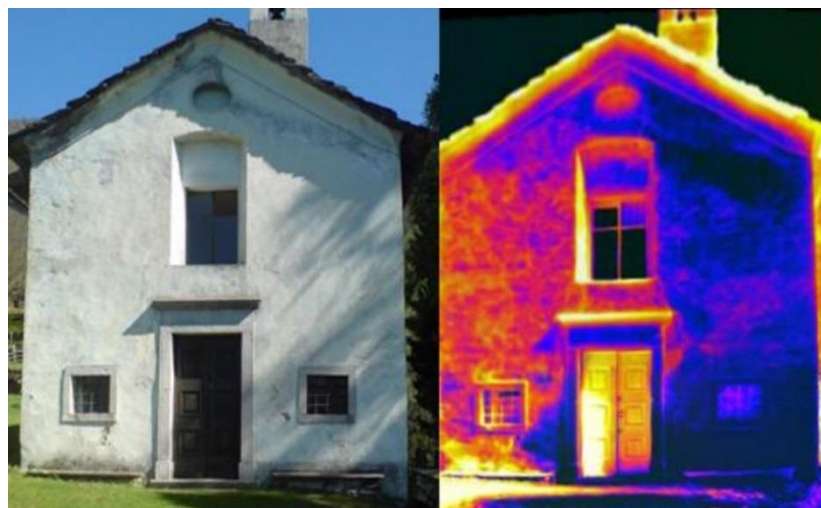
Figure 7. North-West elevation: an example of application of infrared thermography
