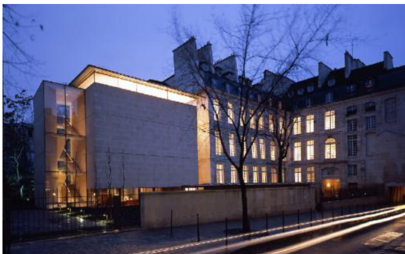
Figure 2. View of the original and added part of the house of photography building
