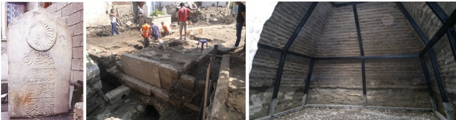
Figure 9. Meddah Baba Tomb archaeological excavation and consolidation works
