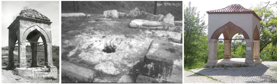
Figure 13. General view of the King's Daughter Mausoleum before the 1963 Earthquake and its view after the earthquake (Bogojević Archive) and after the restoration (Škrijelj, 2017, s. 150)
