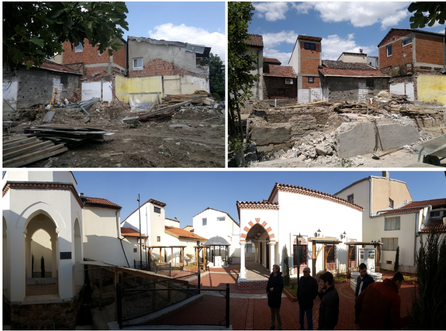
Figure 16. Before and after the project area
