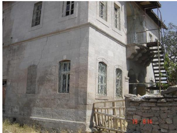
**Figure 8:** *Subsequently Added Stairs And Closed Window (Dülgerler, O.N., 2007)*
