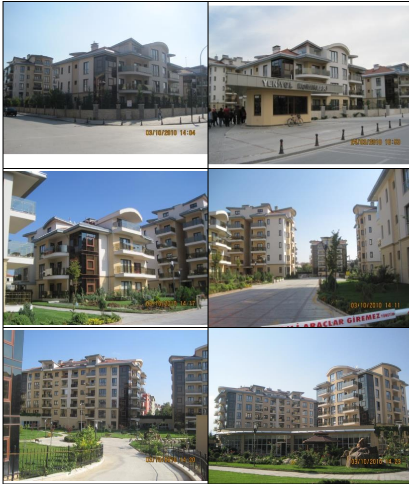
Figure 4. General view of Meram Yeniyoł Residences
