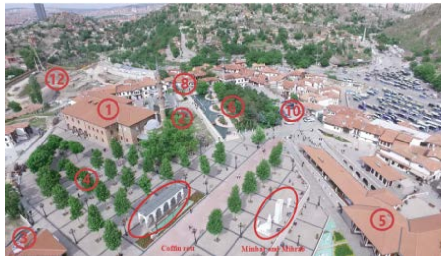
Figure 6. Hacı Bayram Mosque and Its Vicinity
