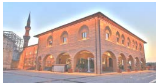
Figure 15. Facade Lighting- Hacı Bayram Mosque
