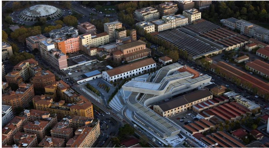
Figure 4. In Zaha Hadid's Maxxi Museum, the phenomenon of difference determines both the building's shape and its relationship with its environment. ( https://www.zaha-hadid.com/architecture/maxxi/ )
