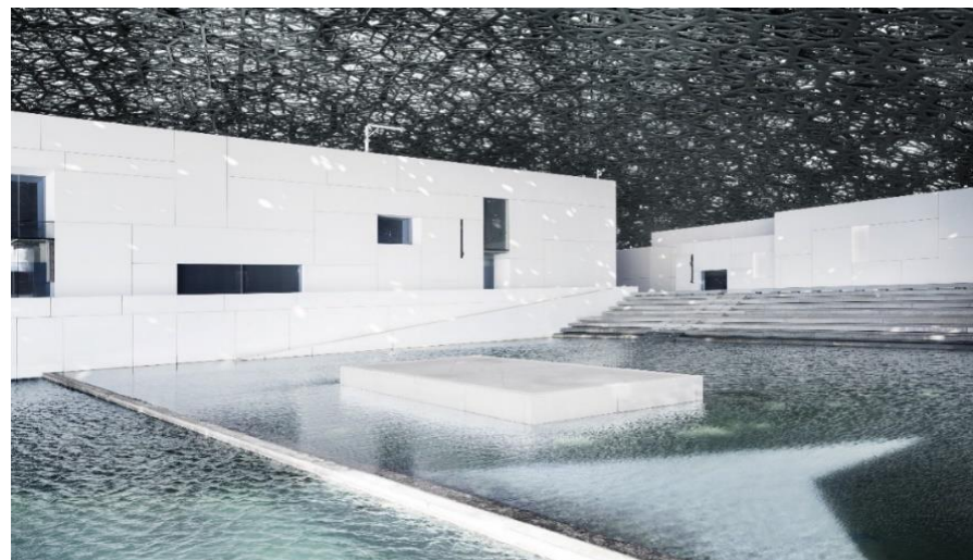
Figure 11. Sunlight filtered in LAD also supports air conditioning system by evaporating water in the internal channels.( Jean Nouveau www.jeannouvel.com/en/projects/louvre-abou-dhabi-3/ )
