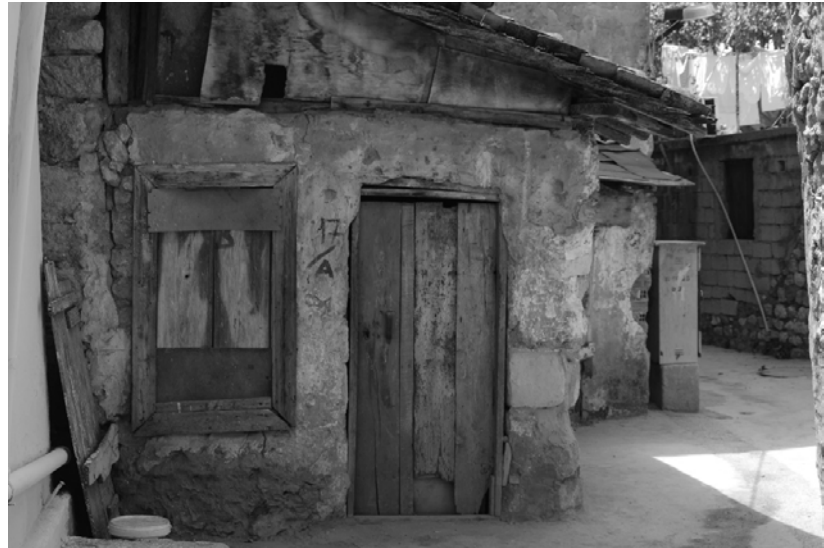
Figure 5. A kitchen and toilet which are still preserving their original relations in a private cul-de-sac (Rıfaioğlu, 2011).
