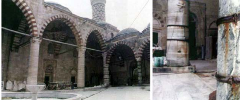
Figure 6. The CL1 column, Üç Şerefeli Mosque (Source: Altınsoy, 1999)
