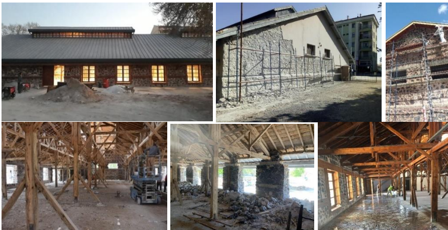
Figure 3. Restoration process of the Karapınar Grain Warehouse (Konya Metropolitan Municipality archive).
