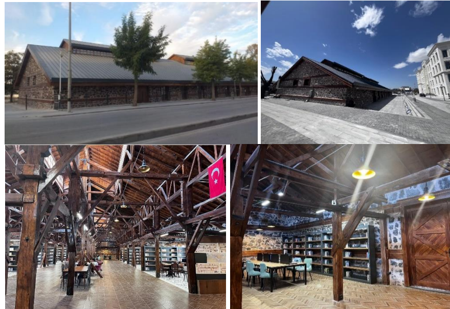
Figure 5. The Karapınar Grain Warehouse after the completion of restoration (Personal archive).
