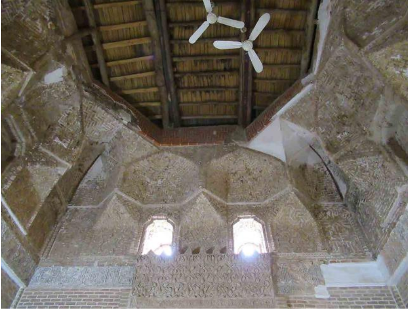
Figure 8. Transitional zone over mihrab in Great Mosque of Marand. Source: Anisi A. (2023) p.318
