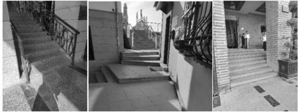
Figure 25. Staircase and Handrail
