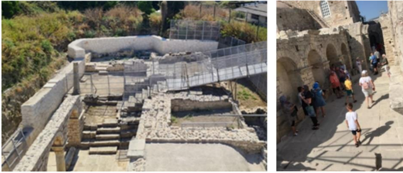
Figure 33. Temporary visitor entrance (AMoCT-PR-4).
