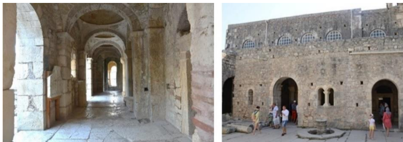
Figure 17. The western outer narthex, Phiale in the courtyard (AMoCT-PR-4).
