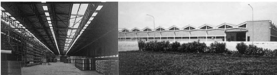
Figure 13. Roof skylights and windows on the façade, which provide natural light to the interior (Boysan, 1997)
