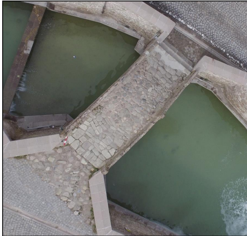
Figure 6. Aerial photograph of the Mısırlıoğlu Bridge.
