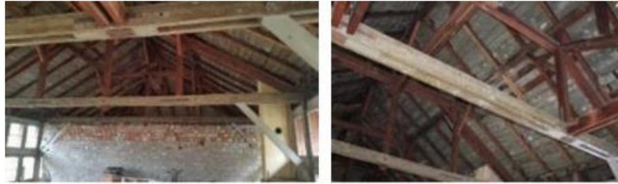
**Figure 7.** Wooden trusses and beams on the roof of the registered structure (Ankara Metropolitan Municipality Culture and Nature Department Archive, 2023)
