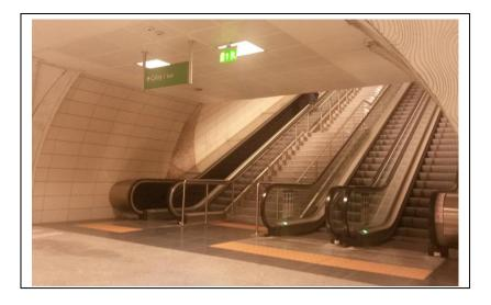
**Figure 5.** Detectable warning surfaces are used at initial and final steps of stairs and escalators.
